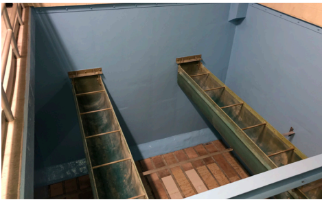
Filter cell completed with coating and filter underdrain installation
