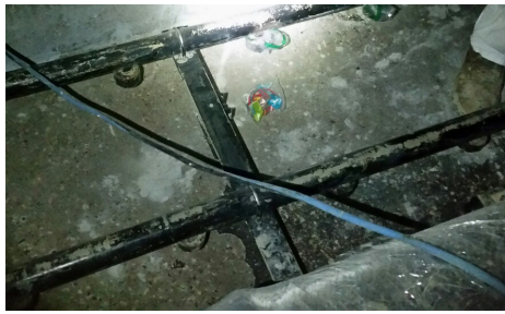
Completed preparation for the installation of new filter underdrains
