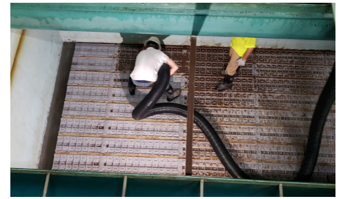
Completing filter media removal for the filter underdrain visual inspection
