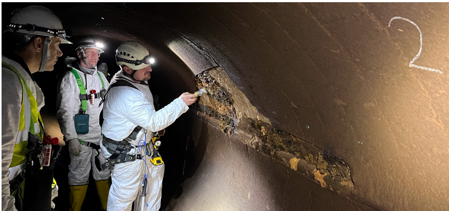
USG employees inspect a water treatment plant.
