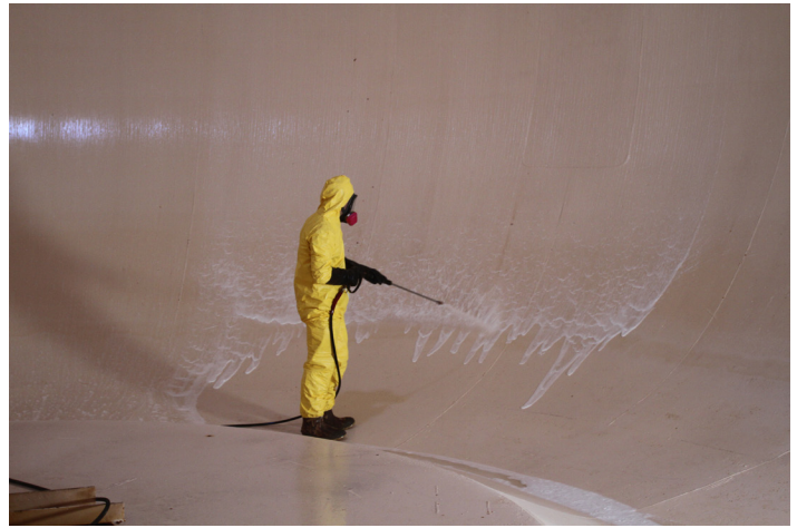
A USG employee cleans a steel water tank.
