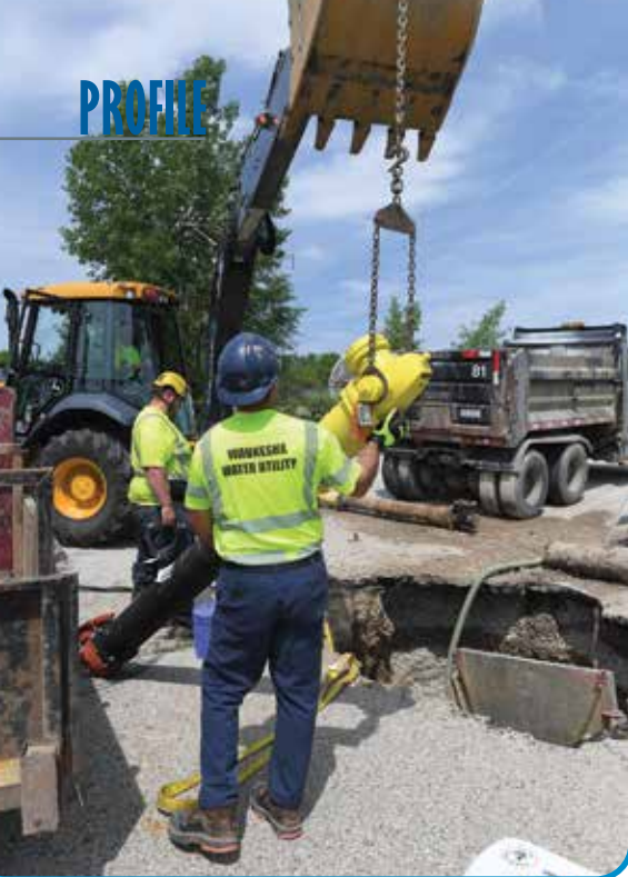
Waukesha Water Utility operators Gus Gentekis (foreground) and Gene Lee swing a new fire hydrant into place.
